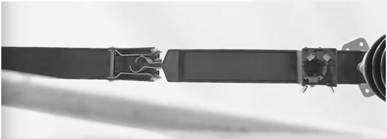
Fig. 18. Correct closing of the disconnector's current path
